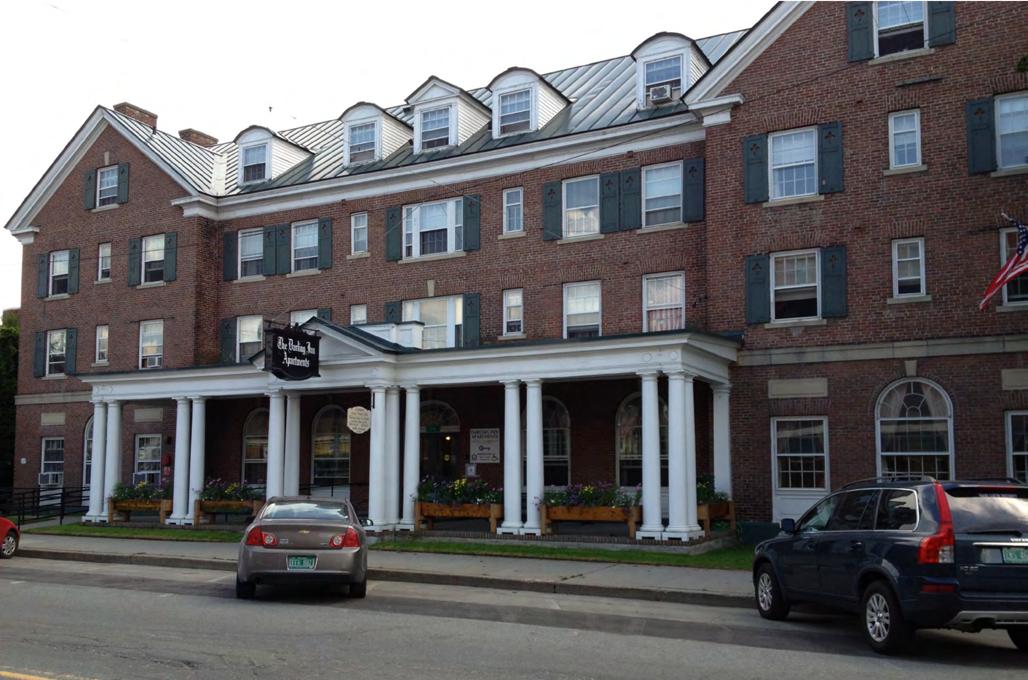
In Lyndonville, RuralEdge is redeveloping senior housing with rental assistance at the Darling Inn, also a site for meals on wheels for the area.
